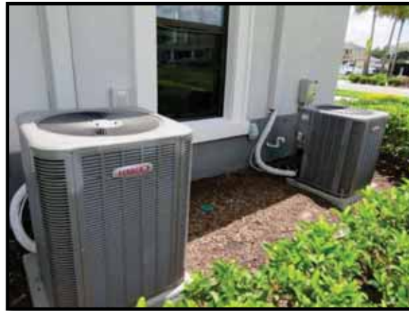
Figure 1 – HVAC Condensers
