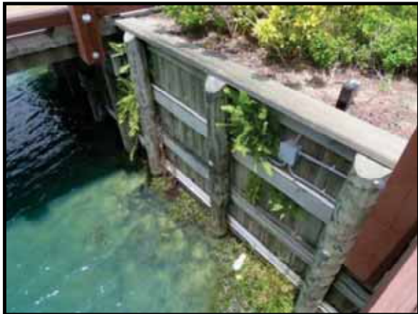
Figure 1 – Wood Bulkhead Retaining Wall
