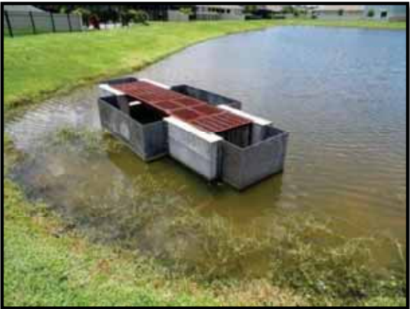
Figure 6 – Stormwater Pond Structure
