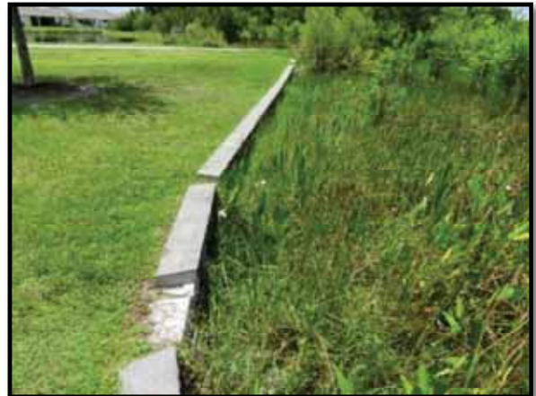
Figure 2 – Masonry Retaining Wall
