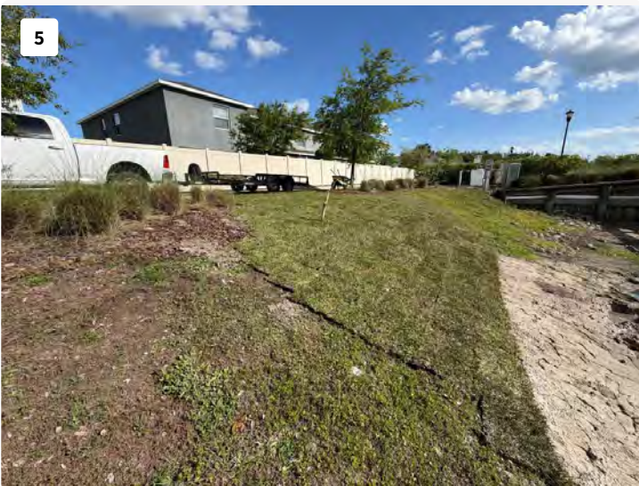
Bank graded to proper 4:1 slope, recommended by SWFWMD.
