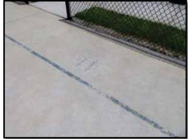
Figure 2 – Exposed Reinforcing
