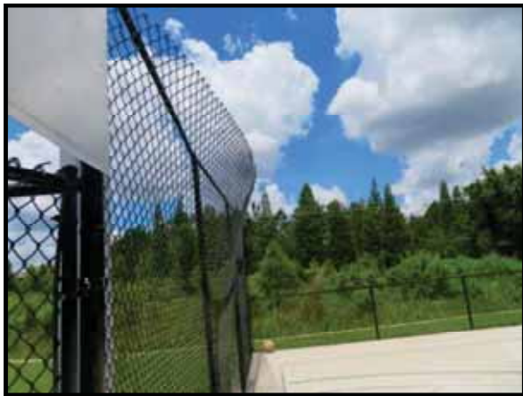
Figure 1 – Basketball Court Fence
